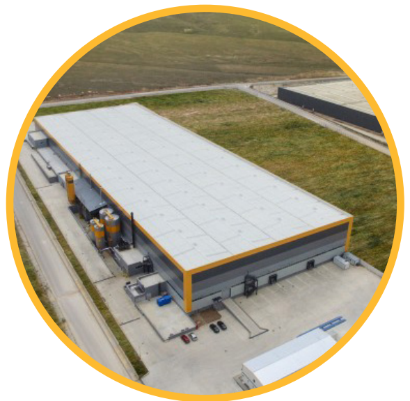
ODE Eskişehir, Turkey Production Facilities
