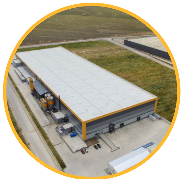
ODE Eskişehir, Turkey Production Facilities
