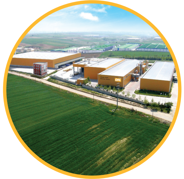
ODE Çorlu/Tekirdağ, Turkey Production Facilities
