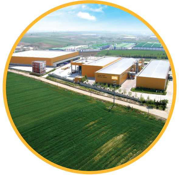
ODE Çorlu/Tekirdağ, Turkey Production Facilities
